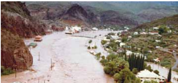
Clifton on October 2, 1983 Courtesy of the Greenlee County Historical Society
